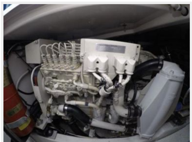
Starboard Main Engine
