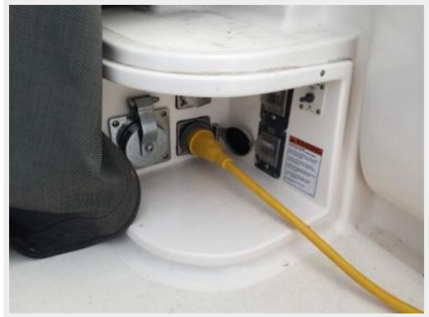
Starboard Shore Power Plug
