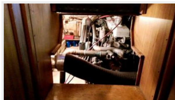
Engine Access from Aft Cabins
