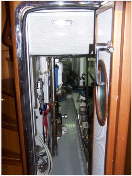
Entry Door to Engine Room
