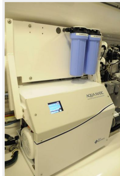
Reverse Osmosis Water MAker
