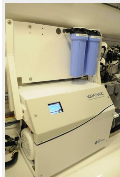
Reverse Osmosis Water MAker
