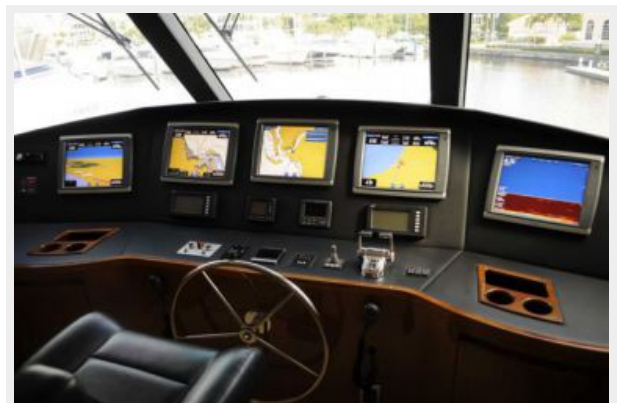
Enclosed Bridge Electronics
