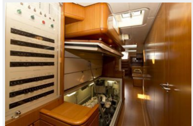
Electric panel and engine
