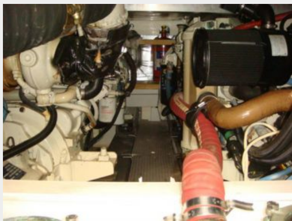
42' Sealine engine room forward
