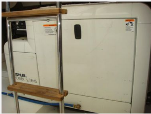
42' Sealine generator soundbox
