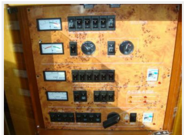
42' Sealine electrical panel
