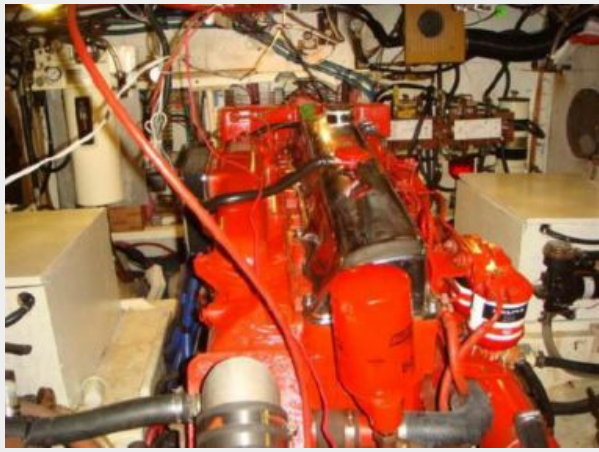
42' Kadey Krogen engine room aft
