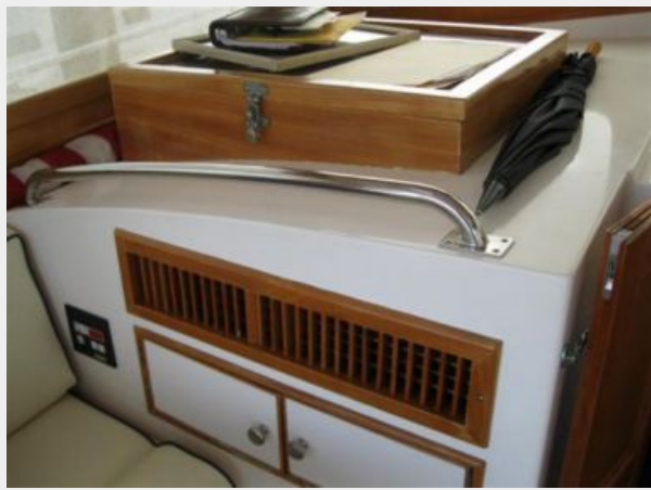
Cockpit air conditioning
