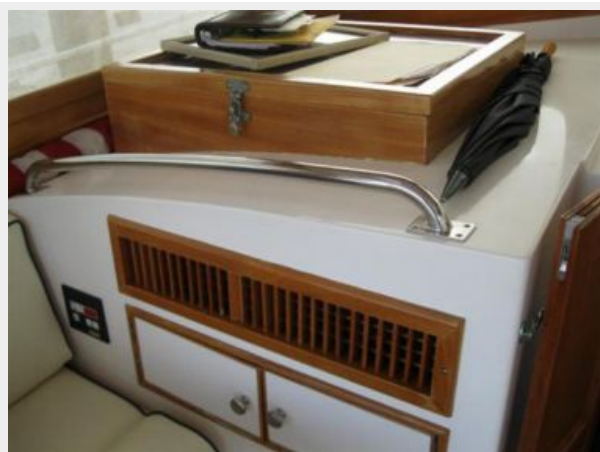
Cockpit air conditioning
