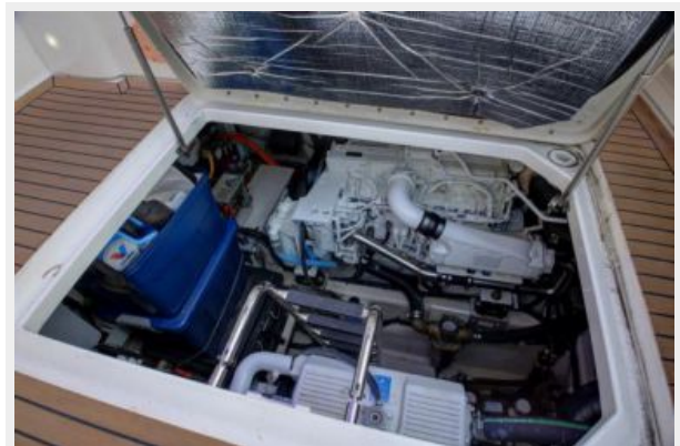
Engine Room / Large Access Hatch
