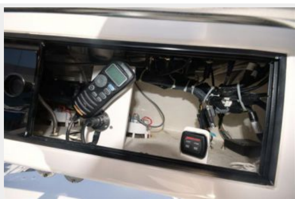
Tower Electronic Box
