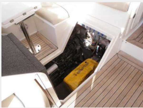
Engine Room Access
