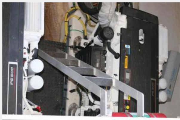
Stairs Going into The Bilge Area
