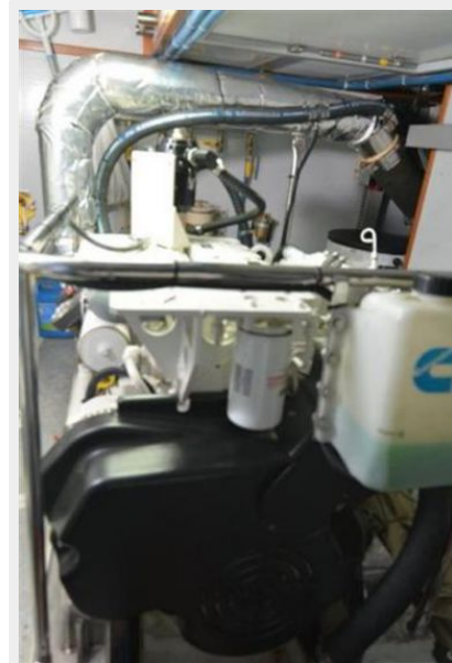
Engine room- Looking aft
