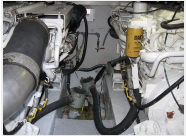
Clean Engine Room
