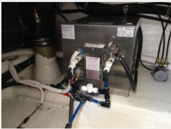
Large 11 gallon water heater
