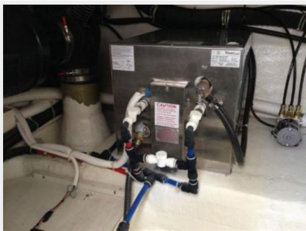
Large 11 gallon water heater
