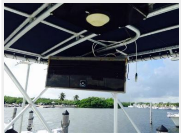
Overhead Electronics Box
