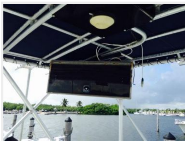
Overhead Electronics Box
