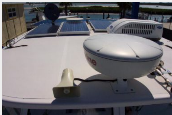
Solar Panels, Helm Air Conditioning, Radar
