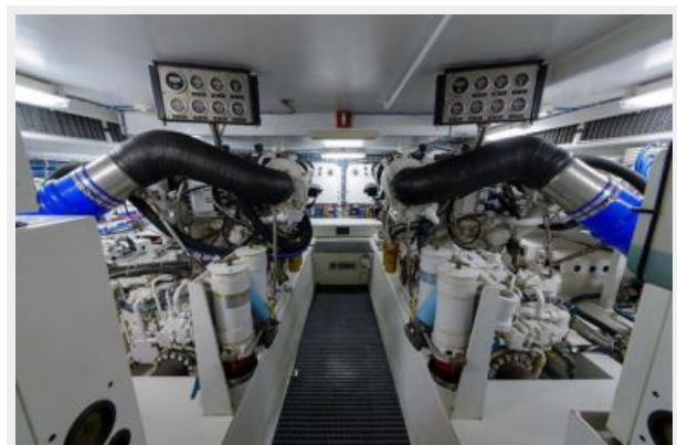
Engine Room Looking Forward
