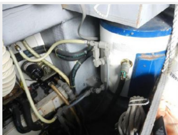
Access Inside Deep Lazarette
