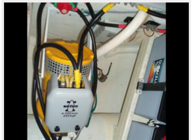
Thruster, Batteries & Charger
