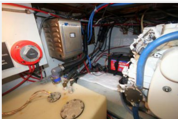
Generator / Battery Charger
