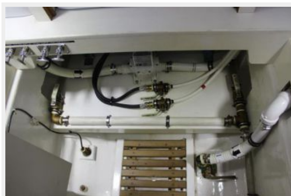
Storage Room - Under the steps down into the galley
