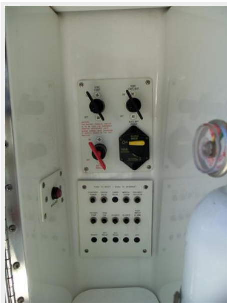
Cockpit electrical panel
