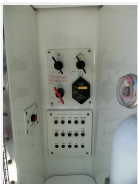
Cockpit electrical panel
