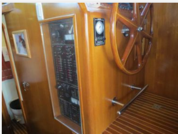
Lower Helm/Electrical Panel
