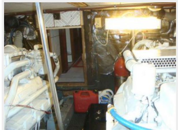
52' Jefferson engine room aft
