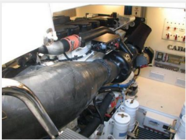
Engine & Mechanical Equipment 3 - Port Engine
