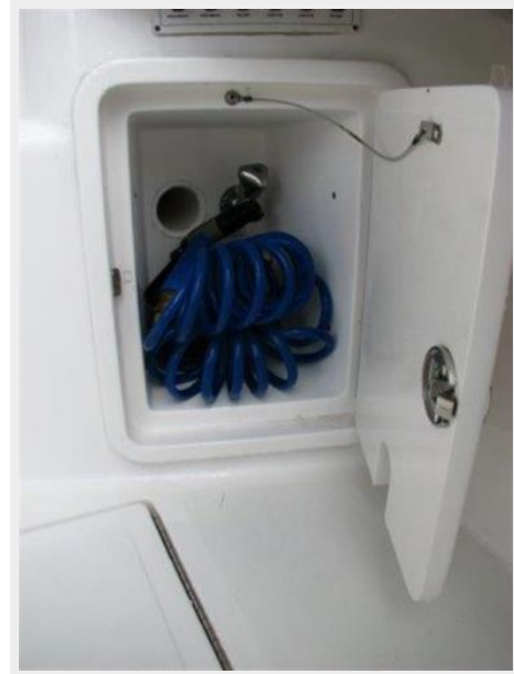
Deck 12 - Deck Wash Down
