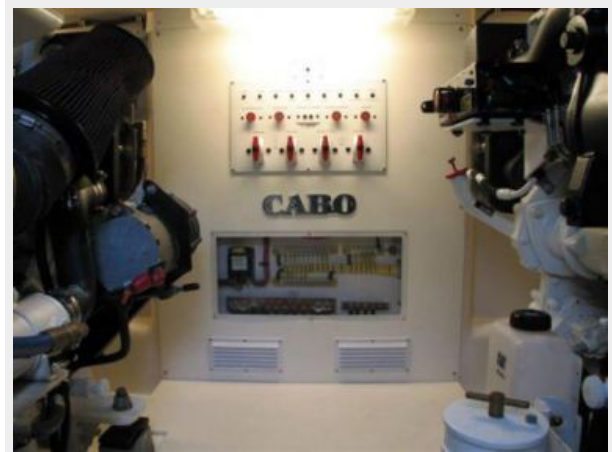
Engine & Mechanical Equipment 2 - Engine Room
