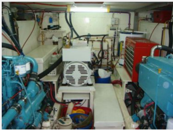
44' DeFever Engine Room Aft
