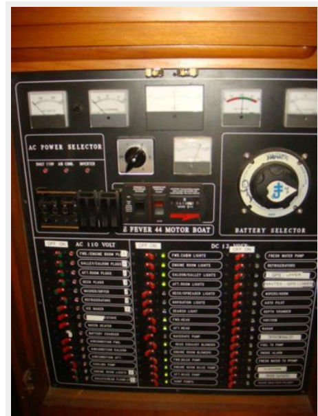
44' DeFever Electrical Panel
