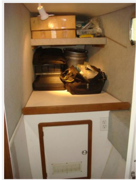
36' Endeavor Starboard Forward Generator Room
