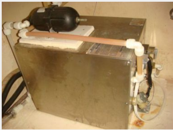
32' Nordic Tug water heater
