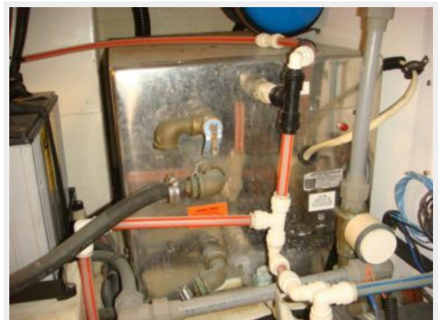
40' Cape Dory Water Heater
