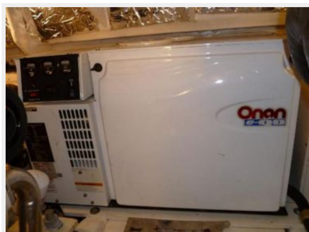
Onan generator w/ sound shield
