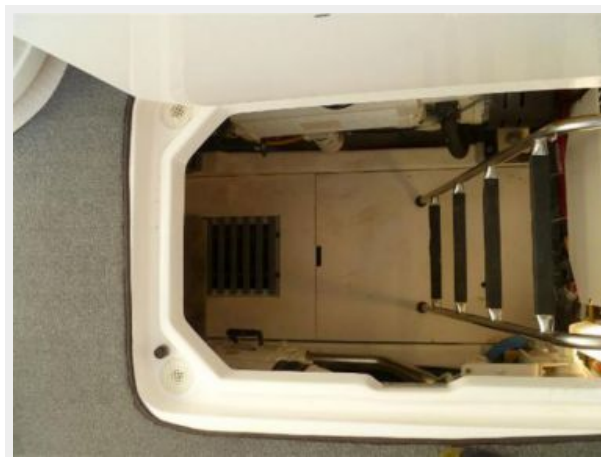
Engine room access
