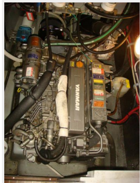
44' Endeavor Starboard Main Engine
