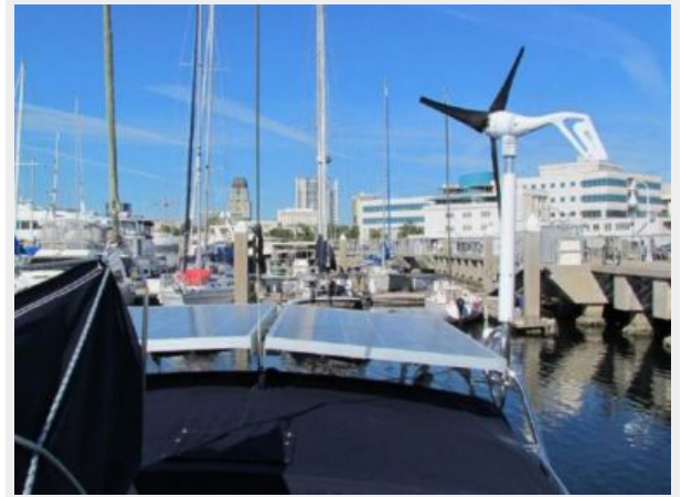
SOLAR PANELS & WIND GENERATOR
