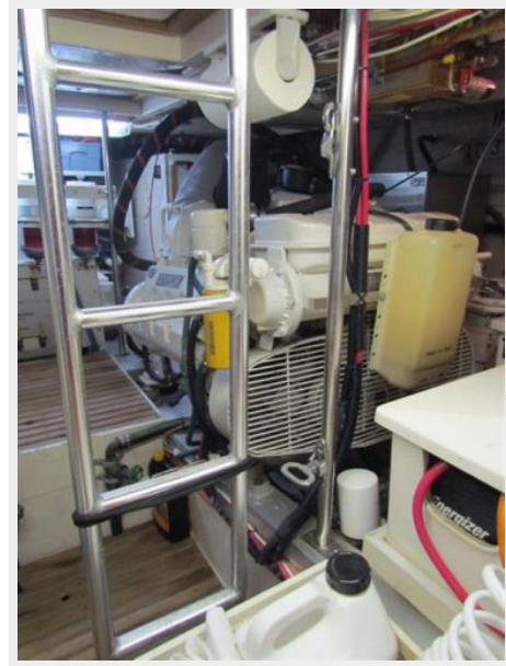
Engine Room Starboard
