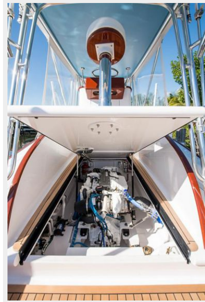
Engine Room Access
