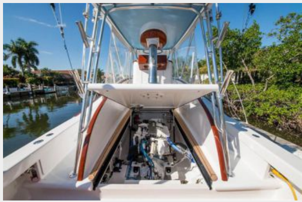
Engine Room Access
