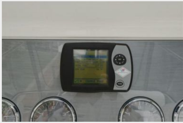
Bridge Helm Electronics
