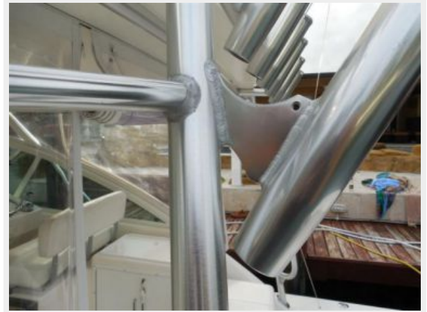
Tower Metal Condition
