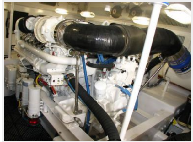
Engine & Mechanical Equipment 3 - Starboard Engine
