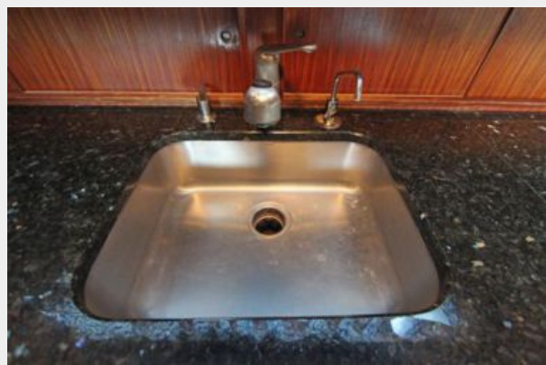
Stainless sink w/disposal
