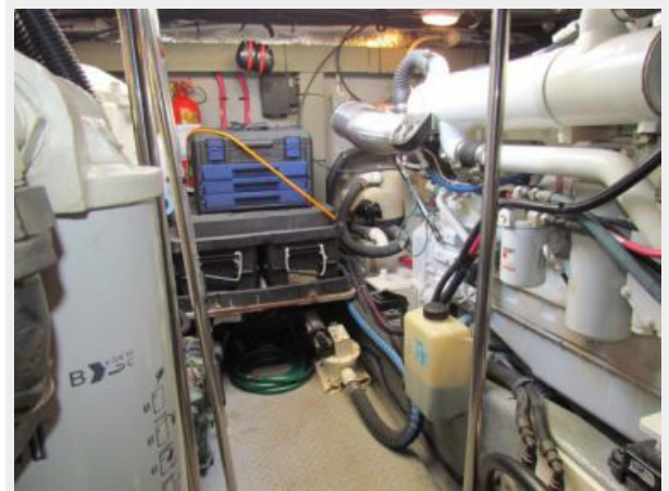
Engine Room Forward
