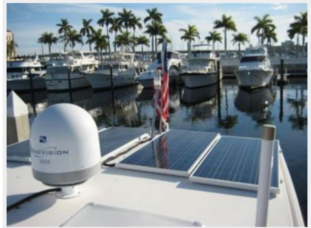
Four 110watt Solar Panels, Tracvision
