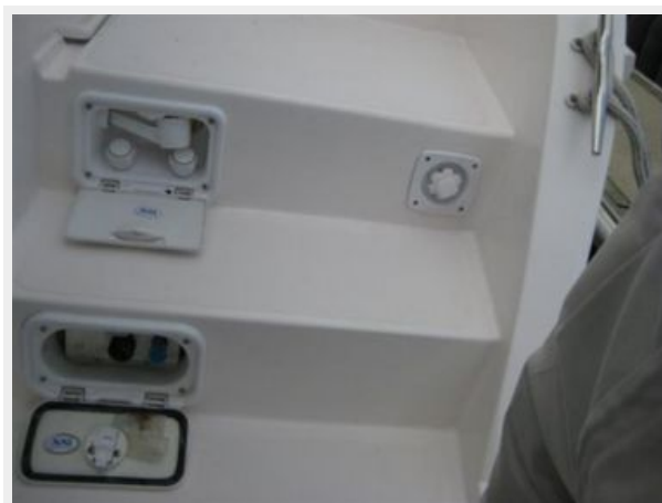
Exterior Shower, Compressor Outlet
