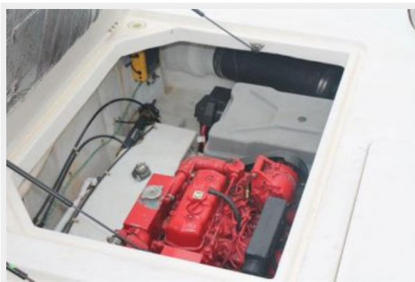
8.0 KW Westerbeke Generator
