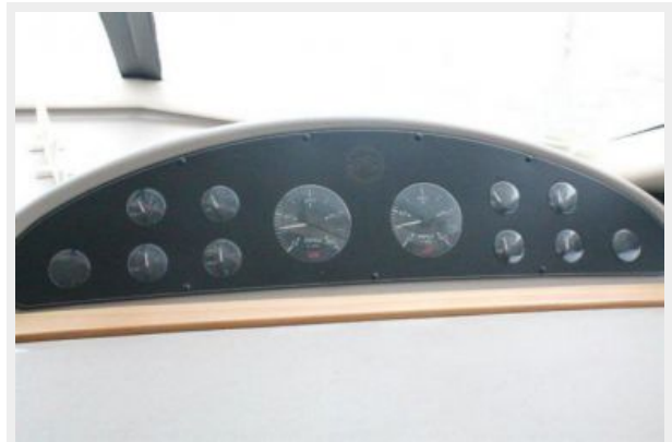
Lower Helm Engine Instrumentation
